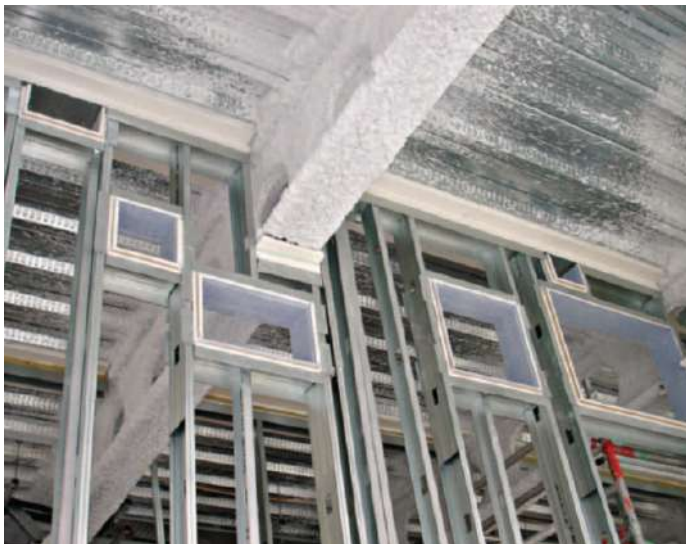
Figure 10 Preprepared openings in a drylined partition (note spacings between openings may differ)
